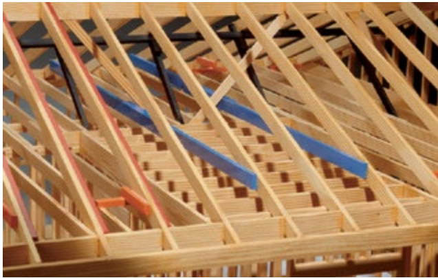
This picture shows 3 different methods of reinforcement, shown in red, blue and black bracing systems
